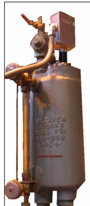
Figure 1-4 Replacement sensor on legacy LM water column
