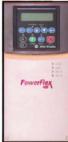
Provides variable speed output to the burner's Combustion Air Fan blower motor for the purpose of improving boiler efficiency and reducing electrical energy consumption.
