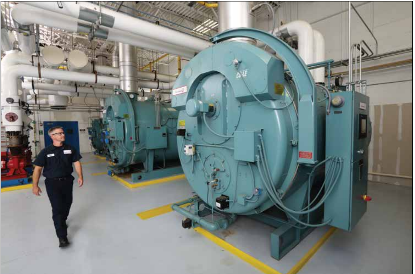
University of Florida Installation of three CBLE firetube boilers
