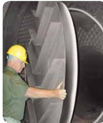
The ICB is unmatched when it comes to serviceability and ease of maintenance. The rear of the boiler includes a davited door which swings completely out of the way to expose a large rear access way (also davited) which
