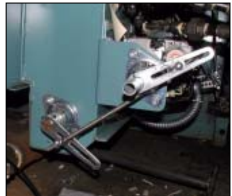
Figure 5-5 Rotary air damper linkage at low fire position
