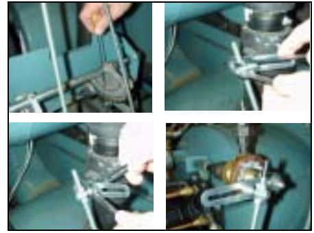
Figure 5-7 Linkage Adjustment
