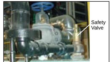
Figure 1-9 Safety Valve
